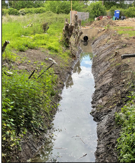
Picture 11 Shermore Brook flow from the site as it exits from under third party land known as ‘Deacons’
