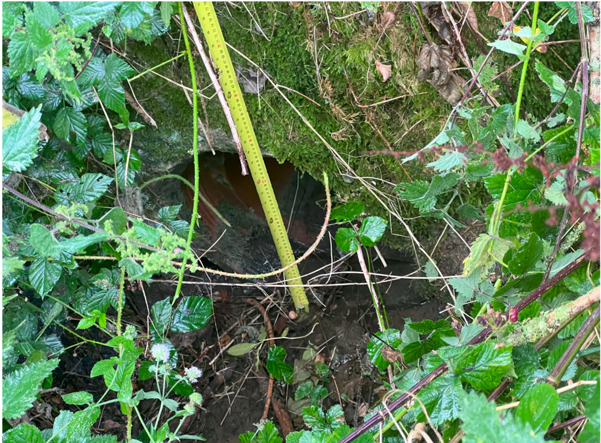
Picture 5 Close up image of Culvert from Western Watercourse passing under B1256 (Location 4 on diagram) 2
