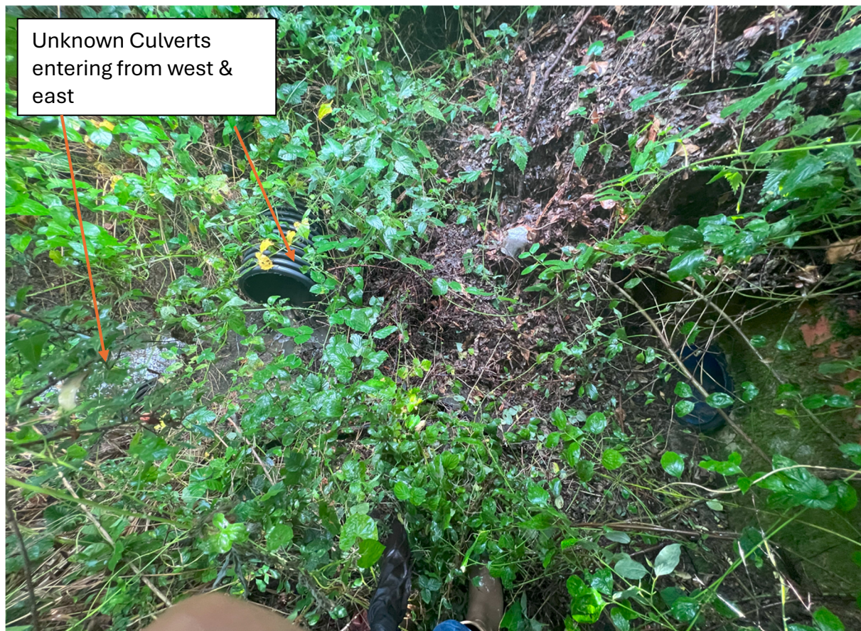
Picture 9 3 x Culverts at Eastern Watercourse (Location 5 on diagram)
