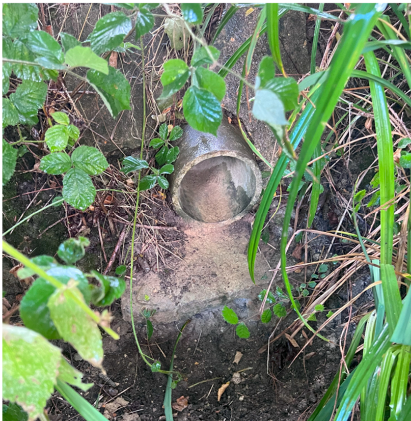
Picture 7 Culvert outfall on western watercourse, arriving from north east angle? (Location 6 on diagram)?
