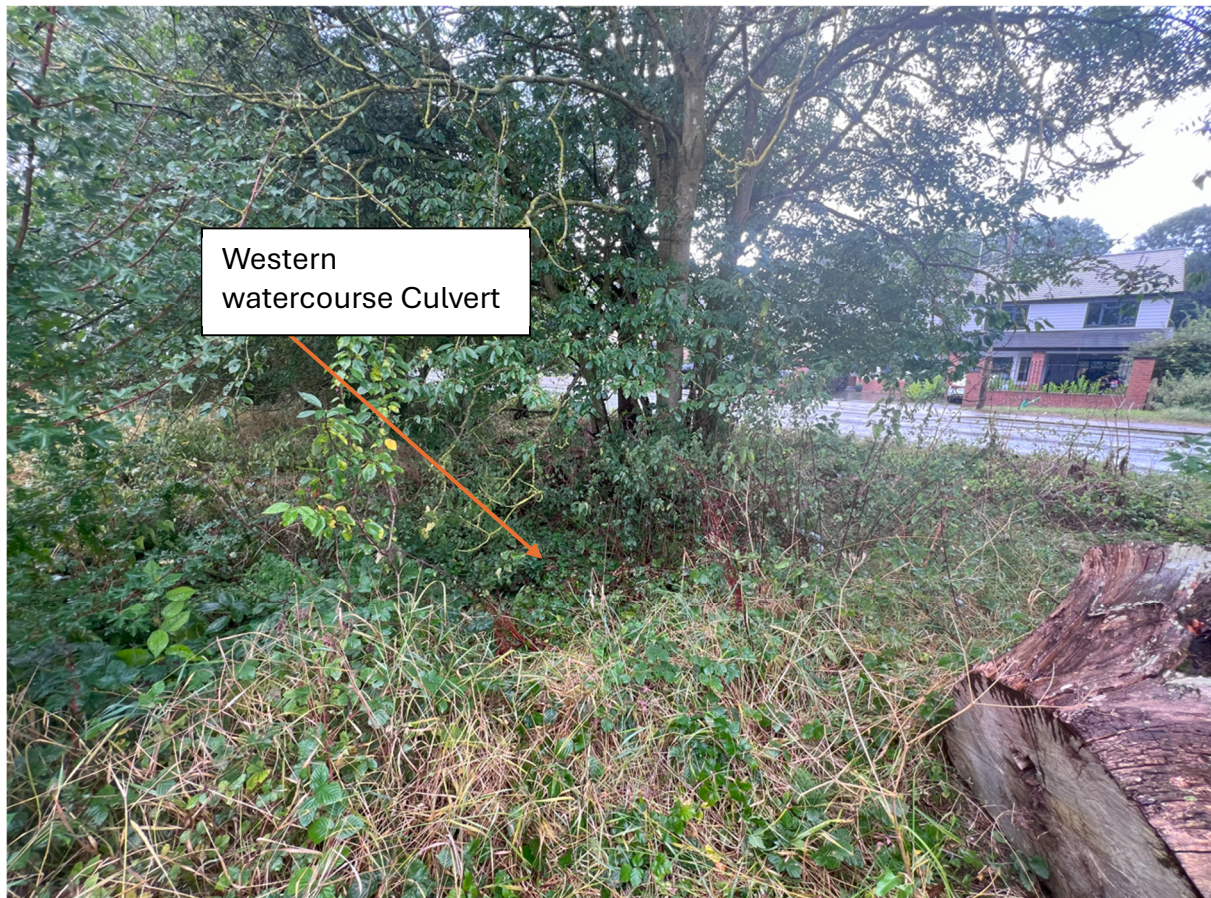
Picture 6 Location of Culvert from Western Watercourse passing under B1256? (Location 4 on diagram)?
