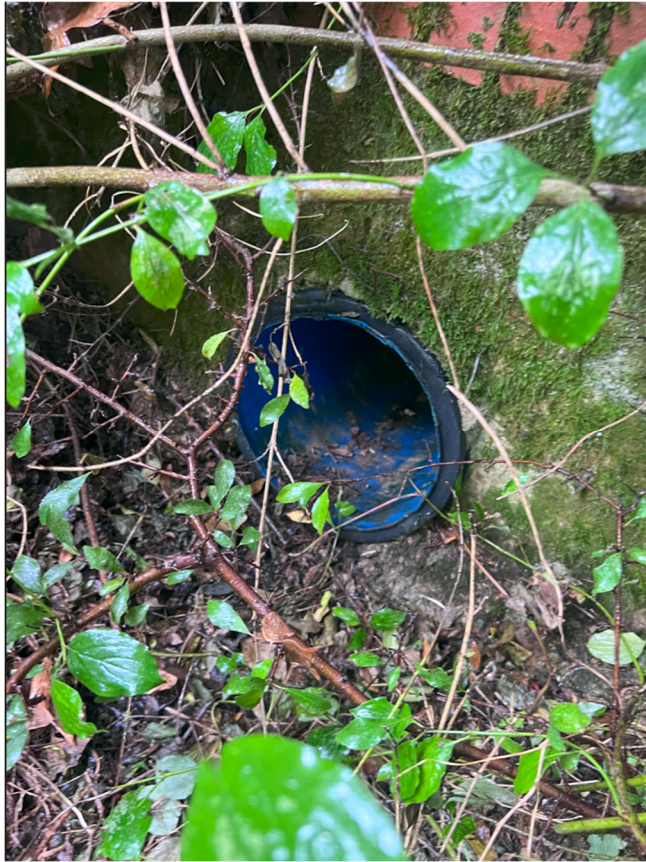
Picture 8 Culvert from Eastern Watercourse passing under B1256 (Location 5 on diagram)
