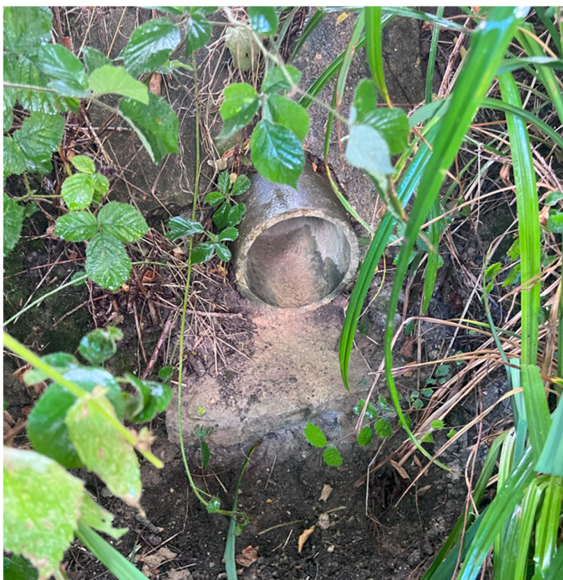
Picture 7 Culvert outfall on western watercourse, arriving from north east angle? (Location 6 on diagram)?
