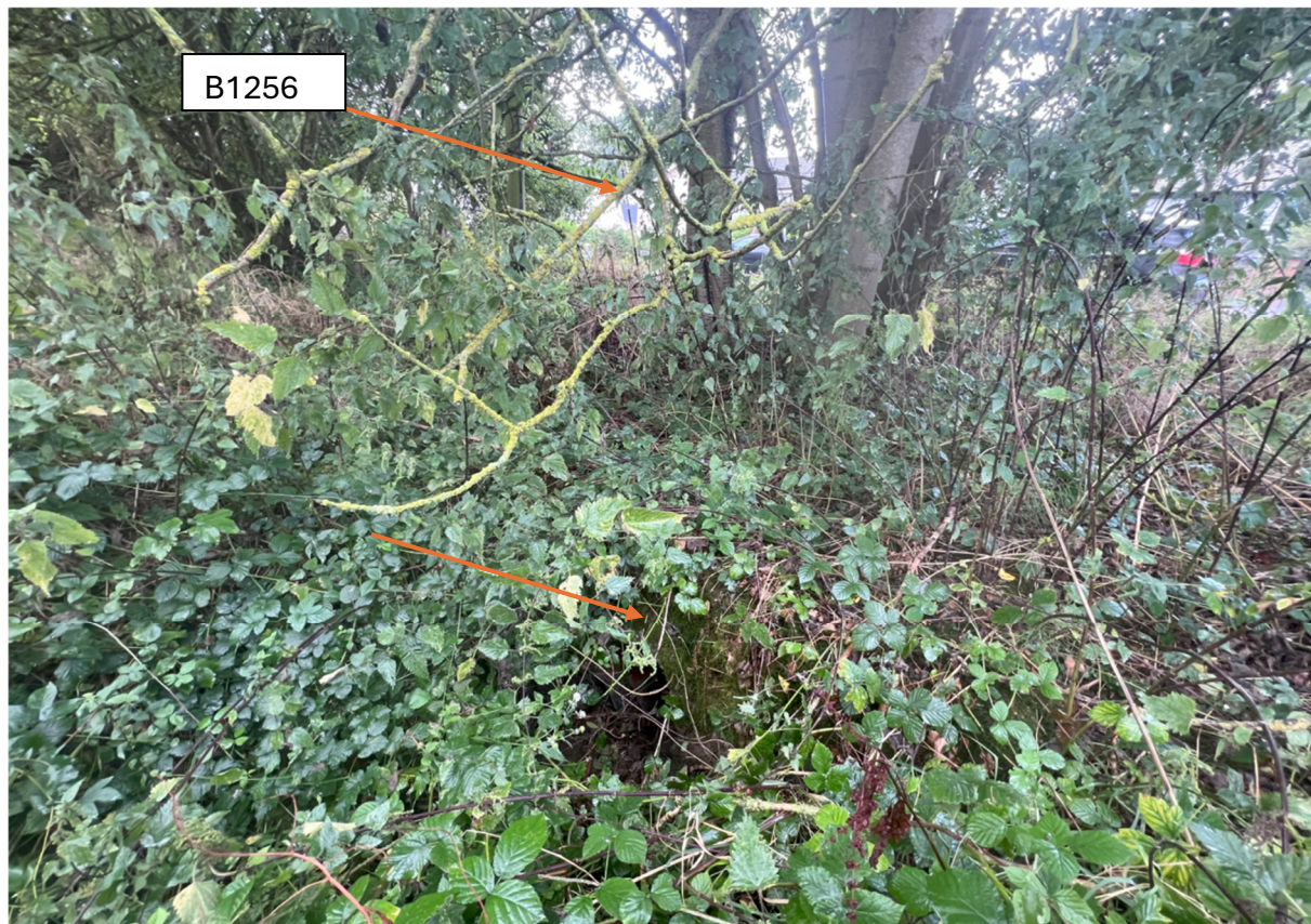
Picture 4 Culvert from Western watercourse passing under B1256? (Location 4 on diagram)?
