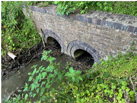
Fig.14 Shermore running through Twin 600mm culverts taking water under the Flichway.
