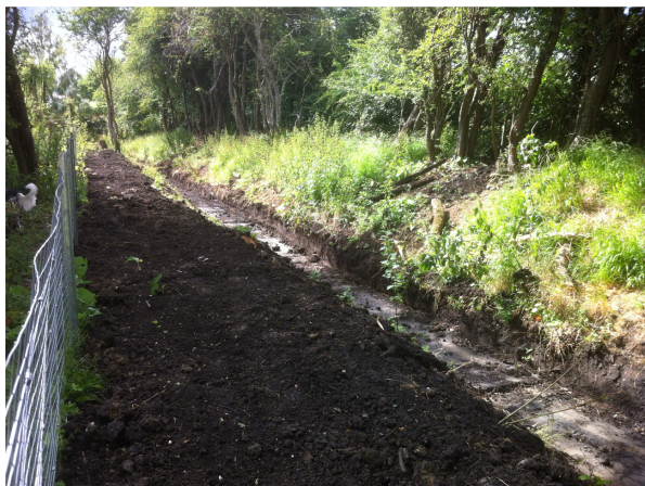
Fig.15 and 16 - Well maintained ditch North of land on South of site between B1256 and Flichway (2017 & 2026). Highway is elevated preventing ANY surface water flowing 'uphill' towards site.
