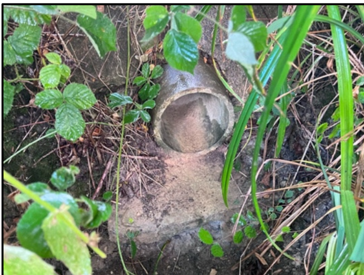
Fig. 5. Land drainage outlet into Shermore Brook (West ditch) central to the site.
