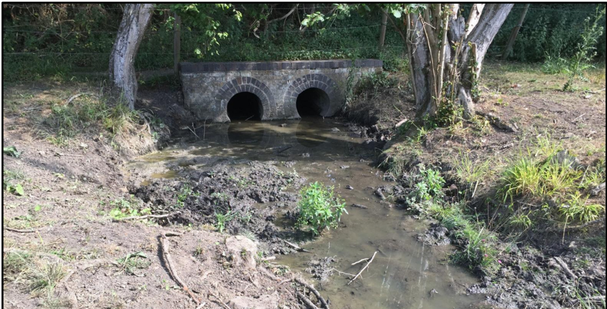
Fig. 9. Shermore 600mm double culvert under Flitch Way – flooding of the SITE is categorically NOT associated with the Flitch Way embankment.
