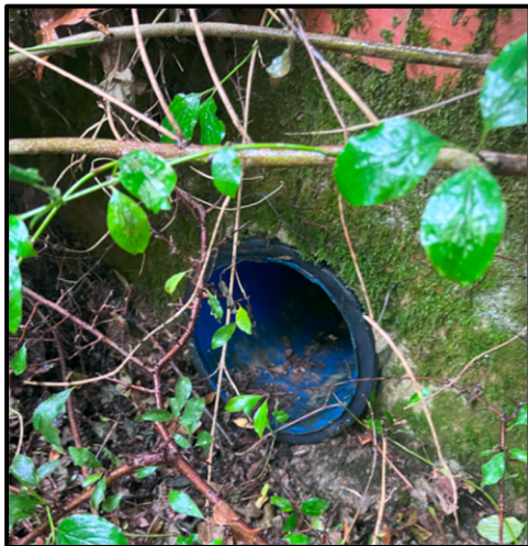
Fig. 7. Close up of culvert with brick header wall at Southern end of East ditch. Route and outfall undisclosed.
