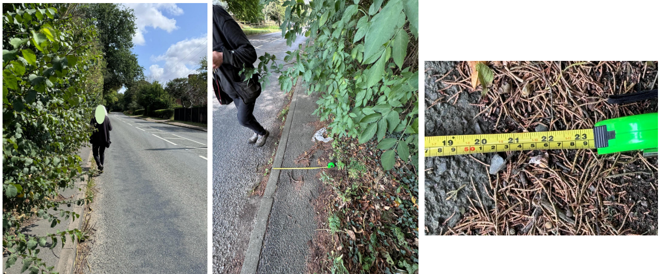
Picture showing pavement West of LNTF (B1256 northern pavement / verge) . Pedestrian forced out on to road. Pavement in this location measures 50cm and is entirely overgrown.
